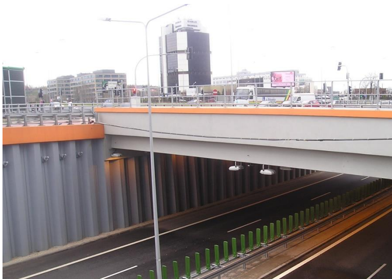
Figure 4. Road viaduct, Kielce
