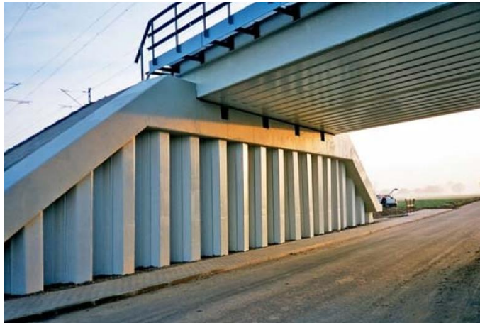
Figure 2. Railway viaduct, Lewin Brzeski
