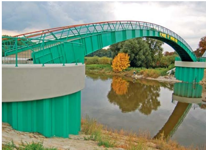
Figure 5. Pedestrian bridge piers, Nowa Sól
